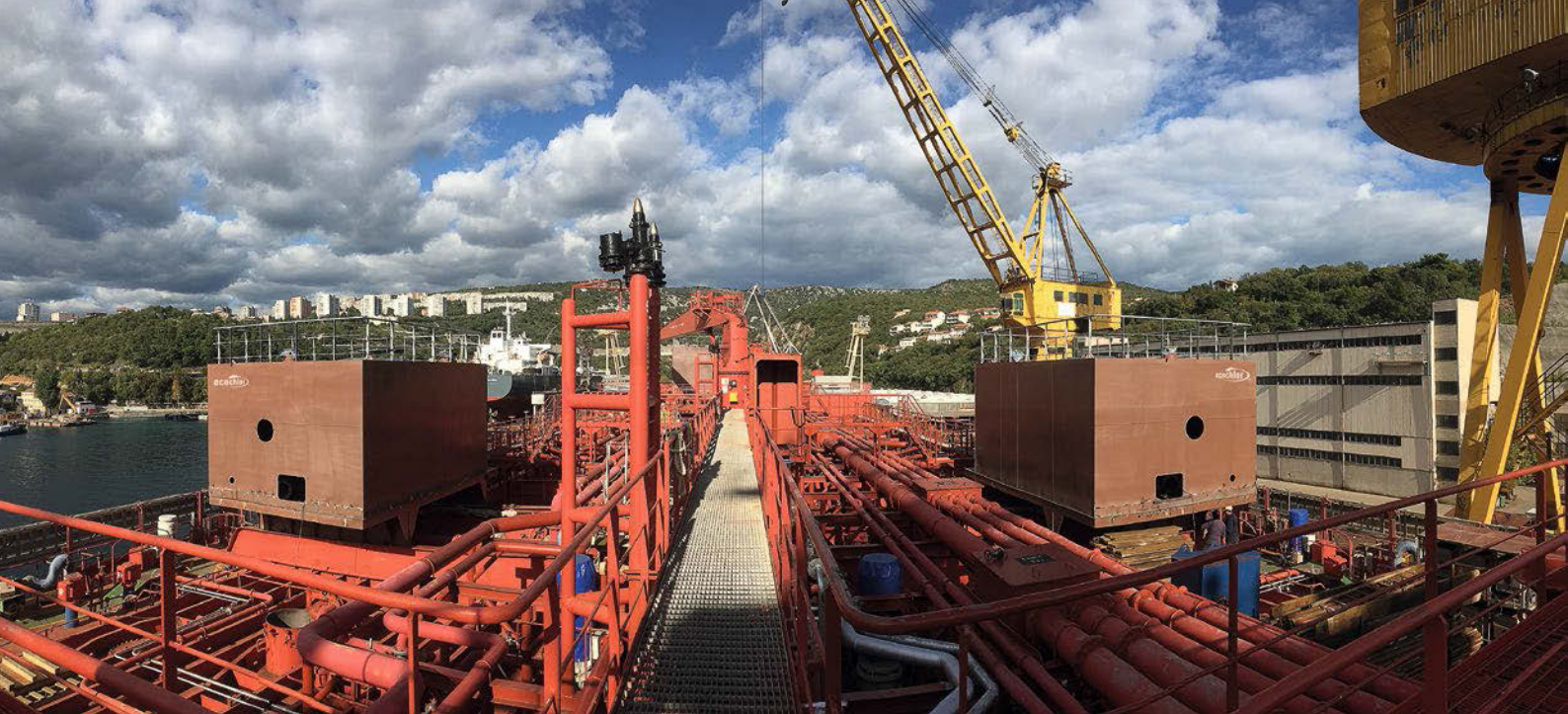
View of main deck and installation of two filter deckhouses
