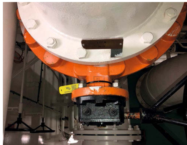
View of the W&O RFID tag and valve Source: W&O Supply Netherlands BV
